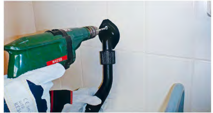
Loch in Platte bohren
